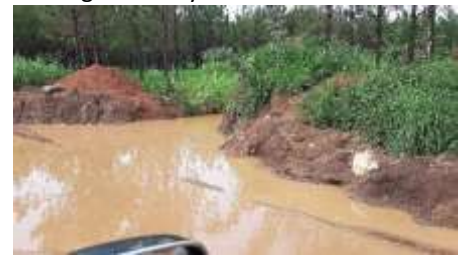
The bypass lane of the Mufulira Road is not really a road in the rainy season
