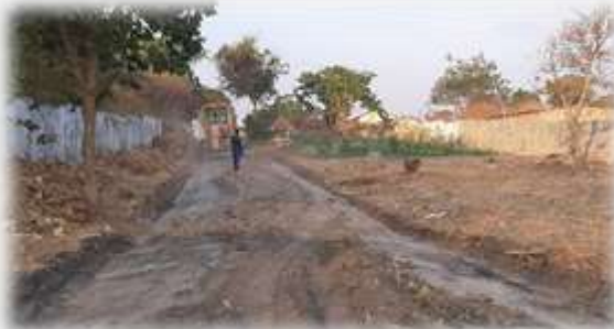
Ready for laterite and shaping
